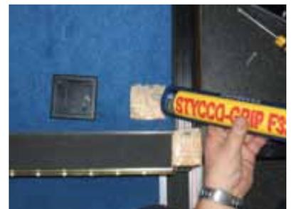
3. Use an adhesive suitable for the substrate
