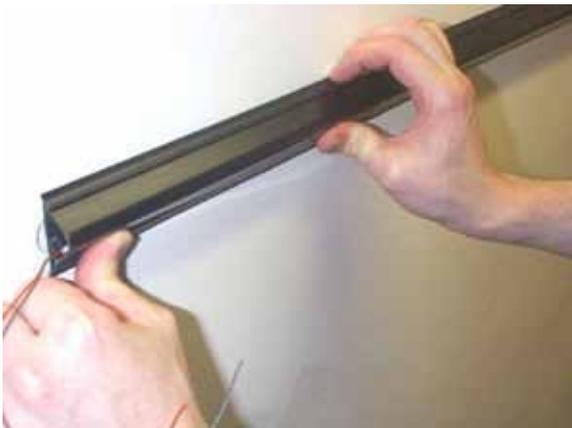
3. The Wall light cover can now be fitted to the base. This simply clips into the base, ensure the clear lens part is on the bottom, allowing the lighting to shine to the floor.
