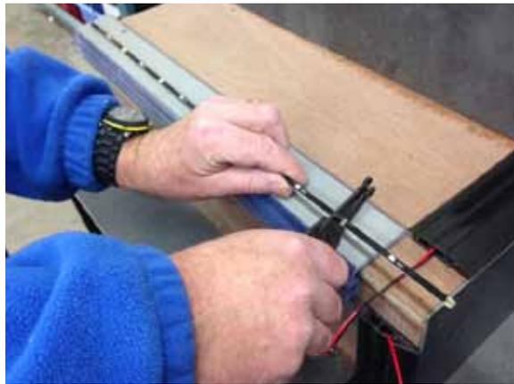
14. Cut circuit board to required length.
