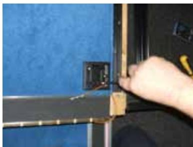
5. Screw base to the floor. NB, **ensure the base is correctly orientated, the embossed letter A indicates how the finished row indicator will appear**
