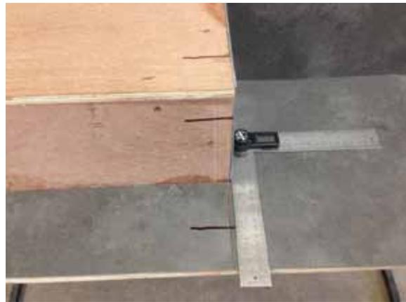
2. Mark below and the back of end caps to determine length of cable Management.
