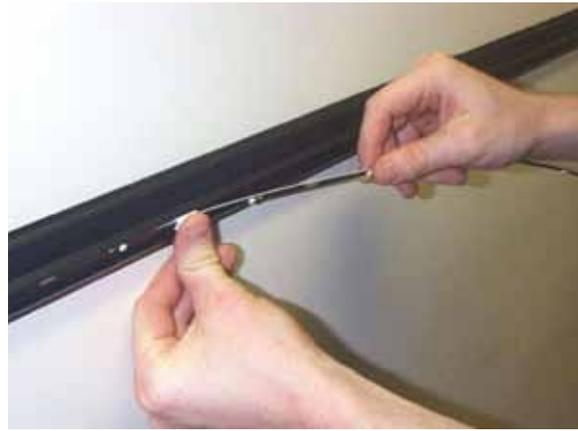
2. Insert the Interlock Advance lighting into the channel in the Wall Lighting housing. Due to the tolerances in the plastics, it may be necessary to use small sticky pads or silicone to hold the lighting in place in the channel. On corners, use the IAVC3 connector as shown on page 9.
