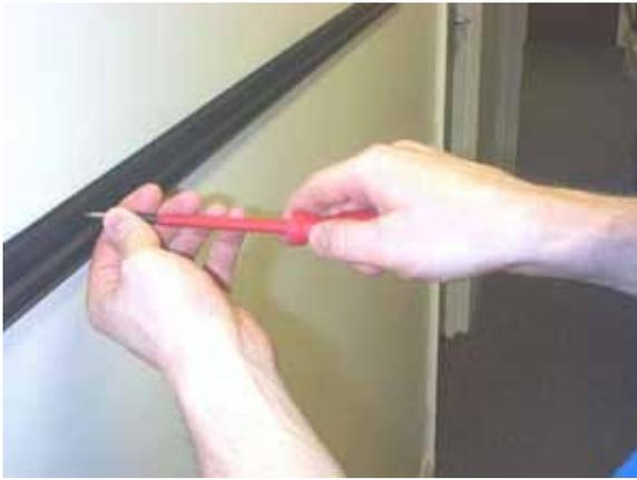
1. Mark the wall in the position where the Wall light housing is to be mounted, drill suitable holes and insert wall plugs. We recommend 3 fixings per metre.
